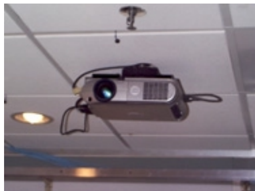
2.1.d – Projector mounted to the ceiling which projects a display onto the opposing wall.
